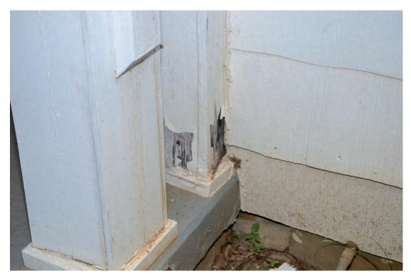
Photo 70. Detail of Pllaster. Note: Paint failure caused splash back and roof flashing leakage.
