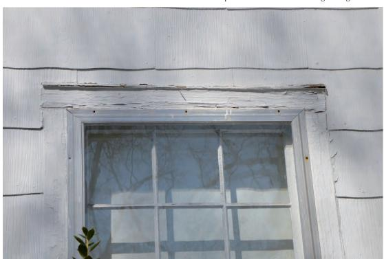
Photo 71. Detail of Window. Note: Paint and caulking failure at lintel.
