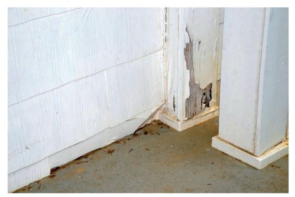
Photo 60. View at Front Porch. Note: Settlement of indicated by compression fracture of cement-fiber shingles at pilaster.
