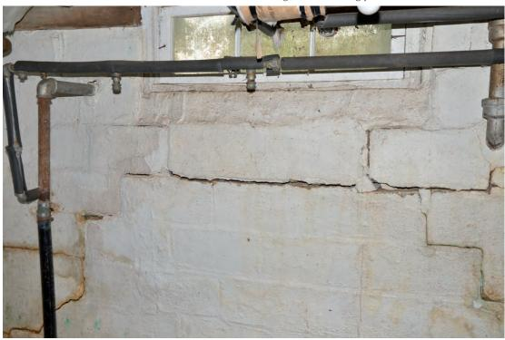
Photo 67. Detail of West Wall at Basement. Note: cracking and wall being pushed out below window.
