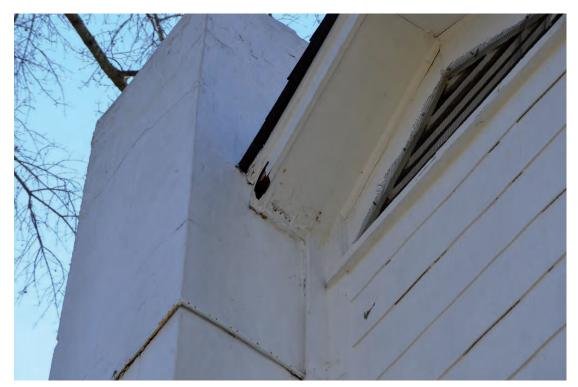
Photo 72. Detail of Eave. Note: Paint and caulking failure caused at chimney.
