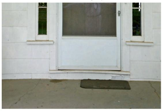
Photo 61. View at Front Entrance. Note: Settlement of door sill and compression fracture of cement-fiber shingles at right corner.
