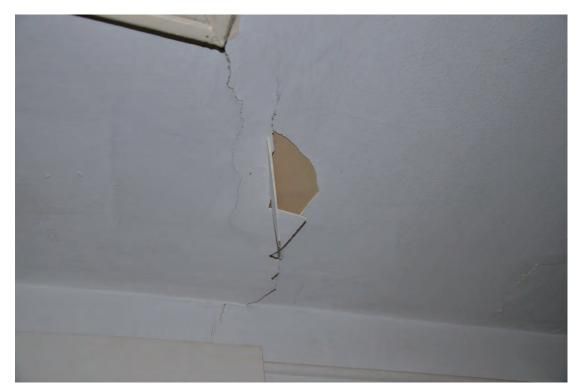
Photo 62. Detail of Settlement Crack
