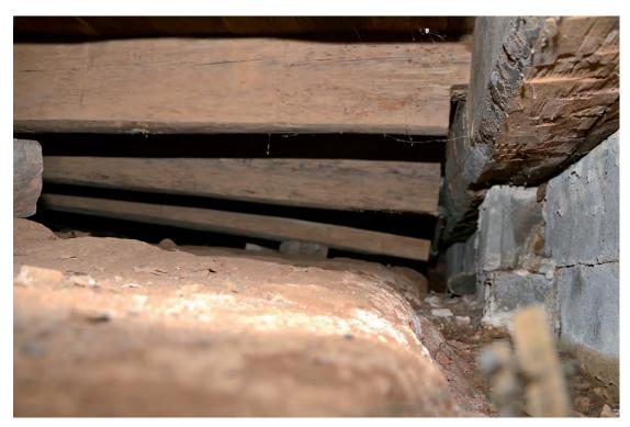
Photo 55. Detail View of Sill at South Facade. Note: Floor joists have slipped away From the sill causing floor system to sag.
