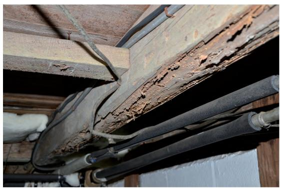
Photo 59. Detail Termite Damage at Floor Joist in Basement.
