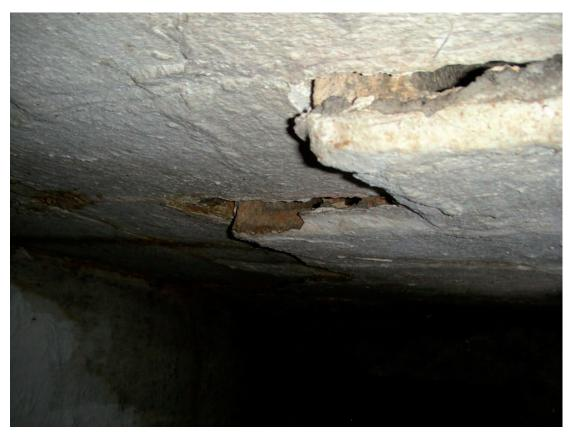
Photo 68. Detail of West Wall at Basement. Note: cracking and wall being pushed out below window.
