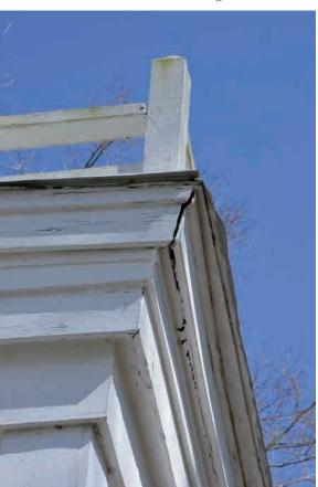
Photo 73. Detail of Porch. Note: Paint and caulking failure at corner.
