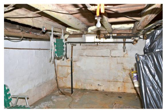
Photo 66. Detail of West Wall at Basement. Note: cracking and wall being pushed out below window.
