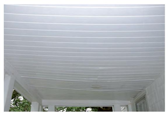
Photo 65. Detail of Porch Ceiling. Note moisture-related damage.
