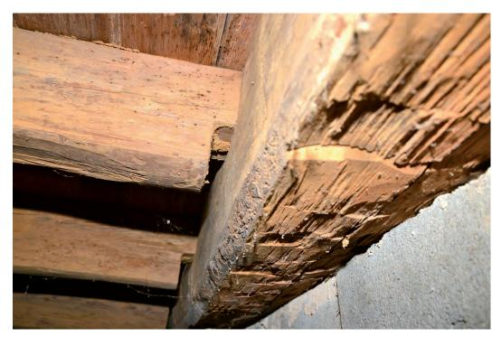
Photo 56. Detail View of Sill at South Facade. Note: hand-hewn sill now Resting directly on concrete masonry unit underpinning (1949/51)
