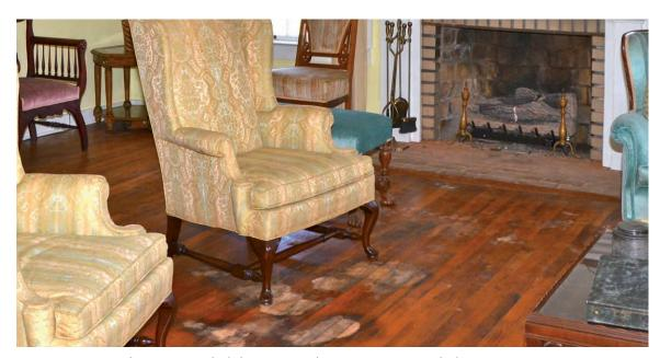
Photo 74. Detail of Flooring at Parlor (Room 103), Detail of Pet Staining.
