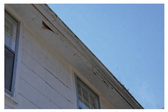
Photo 69. Detail of North Gutter. Note: Paint failure caused by clogged gutters.
