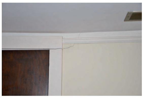
Photo 63. Detail of Settlement Crack, Room 204
