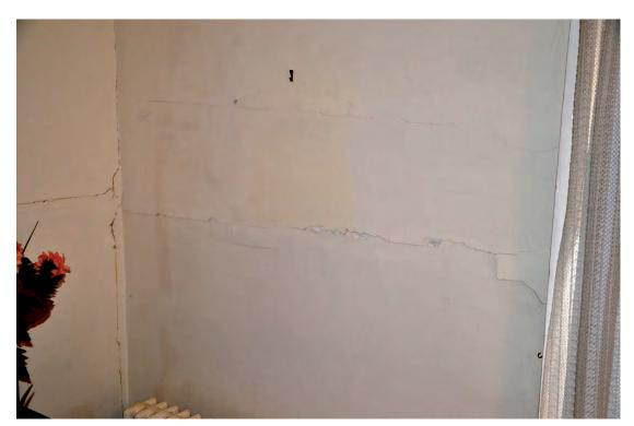
Photo 64. Detail of Settlement Cracks.
